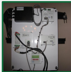
VSD & SWB Upgrade – Retrofit
